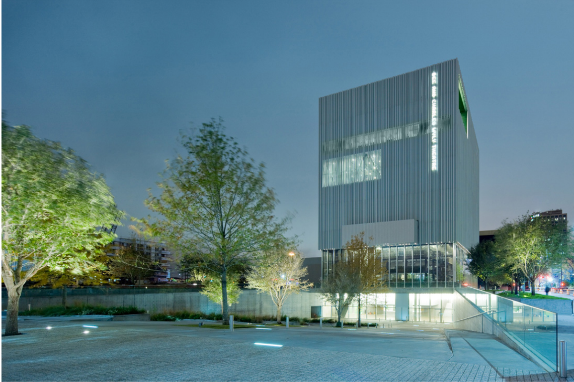
The Dee and Charles Wyly Theatre, designed by REX/OMA (Joshua Prince-Ramus, partner in charge, and Rem Koolhaas), at the AT&T Performing Arts Center in Dallas. Photo by Iwan Baan.
